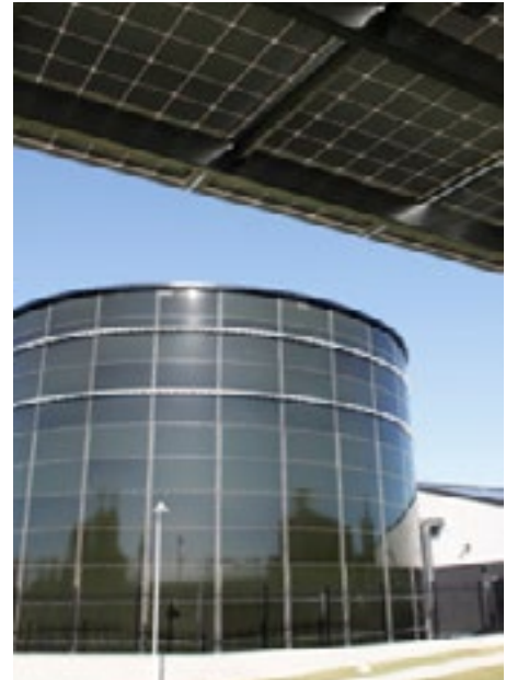
Water battery at UniSC Sunshine Coast campus
