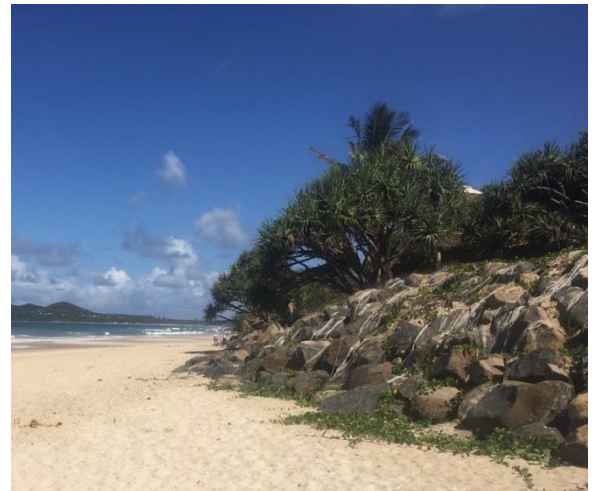
Figure 1: Existing seawall at Belongil Beach.
