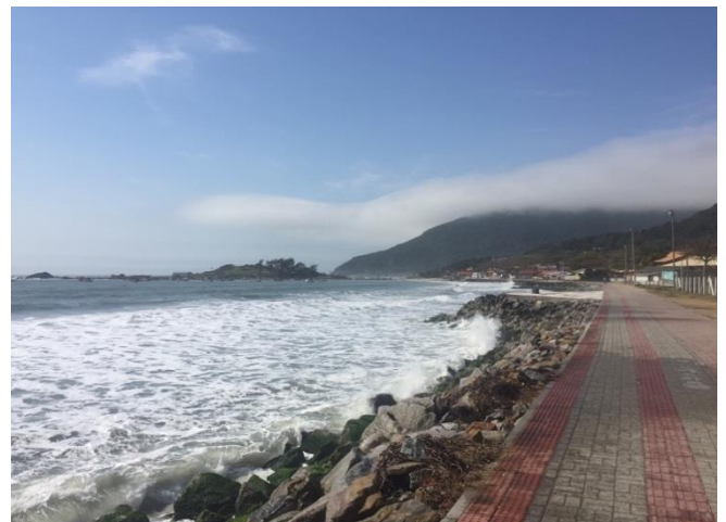
Figure 1: Existing seawall at Armação Beach.
